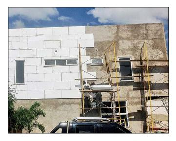
EIFS integrates 3 proven components - a continuous waterproof air barrier, exterior insulation and a variety of textured finish options - into a superior, sustainable wall cladding unlike any other.
